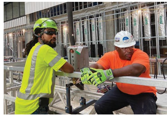
Michael Brown (left), Summit Anchor project manager, sports a high-visibility helmet with an integrated visor while consulting with Tyrone Powers (right), Spider technician, at a project in Washington, DC, in August 2022. Powers is wearing a traditional construction hard hat.
